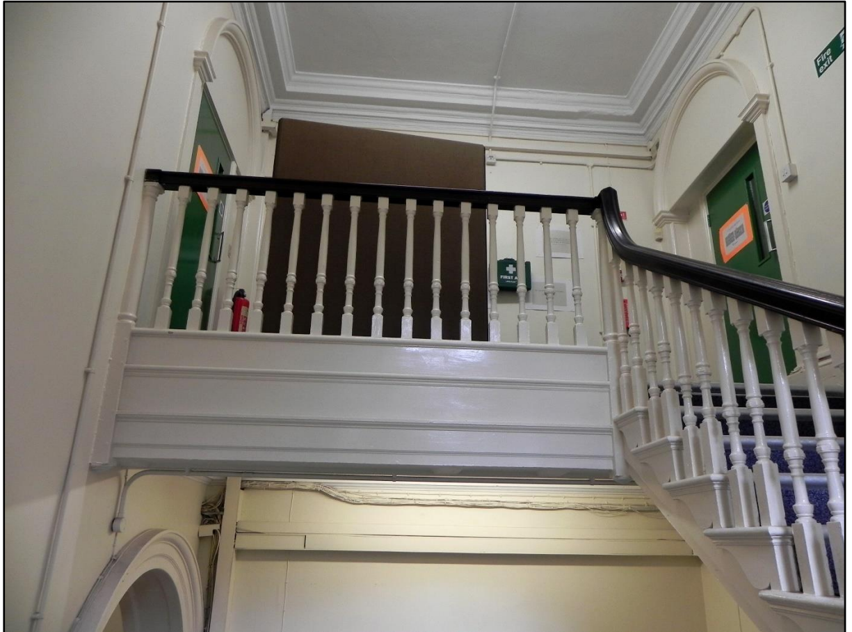
Fig 14 The main staircase showing the landing.
