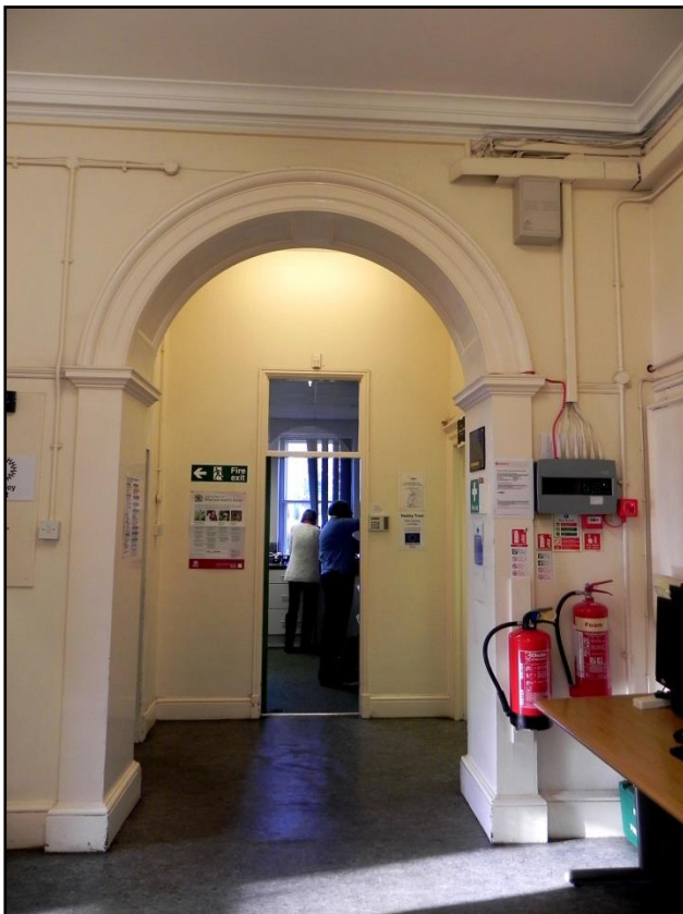
Fig 16 The original entrance to Meersbrook Hall.
