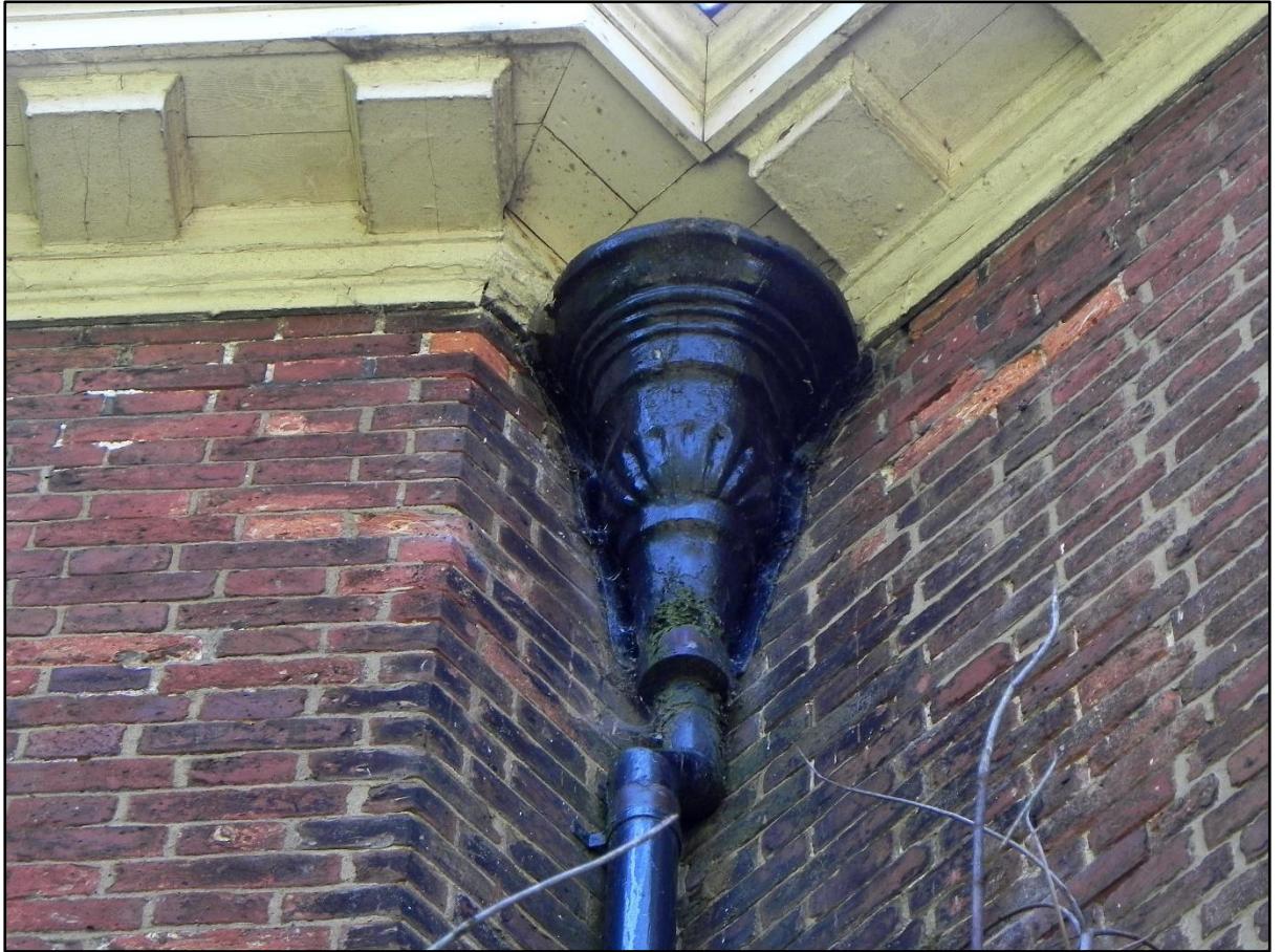
Fig 18 Decorated drainpipe head to the west of the bay window.
