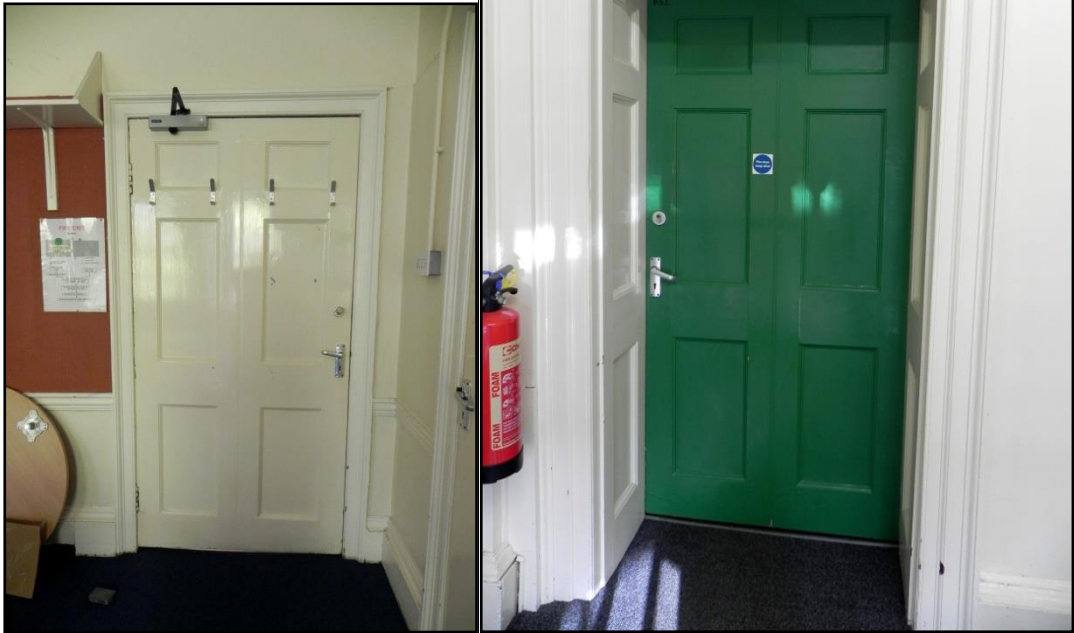
Fig 6 Two of the six-panelled doors.
