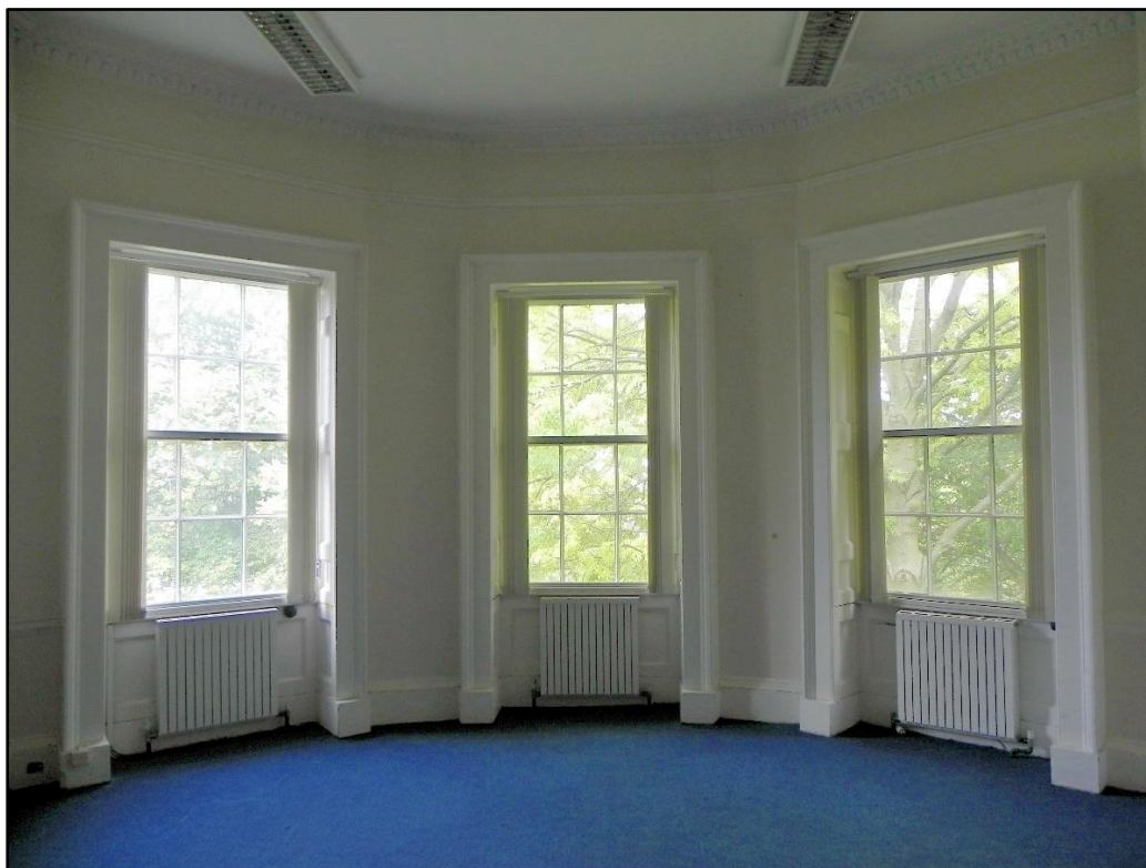
Fig 13 Interior view of the bay window.
