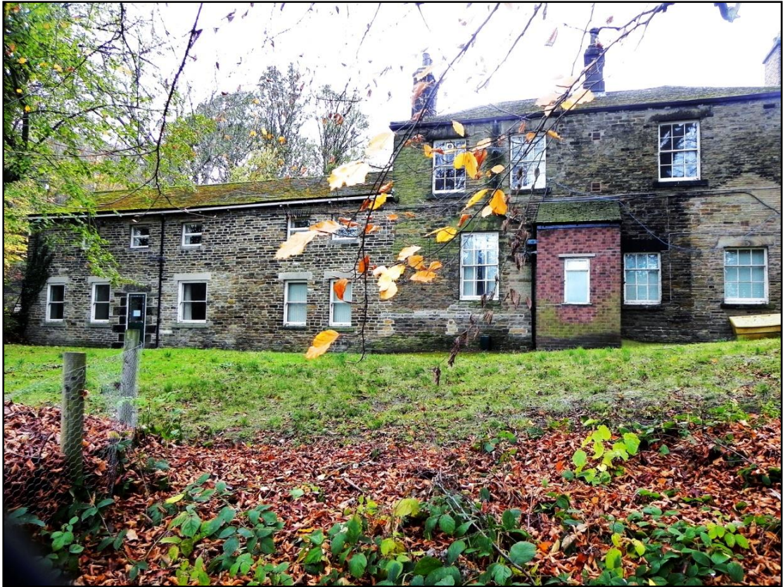
Fig 2 North elevation of the sandstone building.
