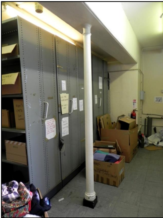
Fig 8 The iron pillar and the retaining beam above.
