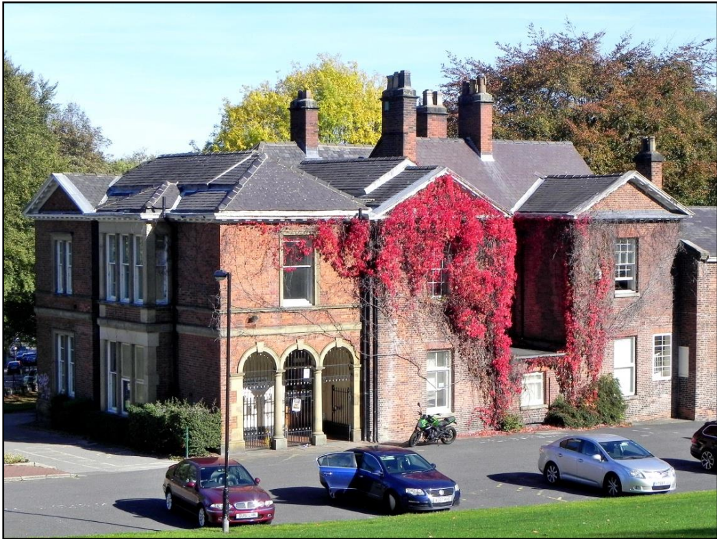
Fig 17 General view of Meersbrook Hall, south elevation.
