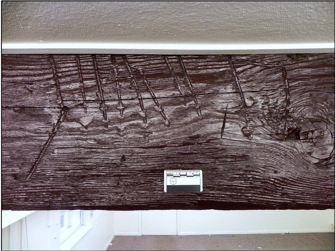
Fig 27 Baltic shipping marks on one of the ceiling beams (group 7).
