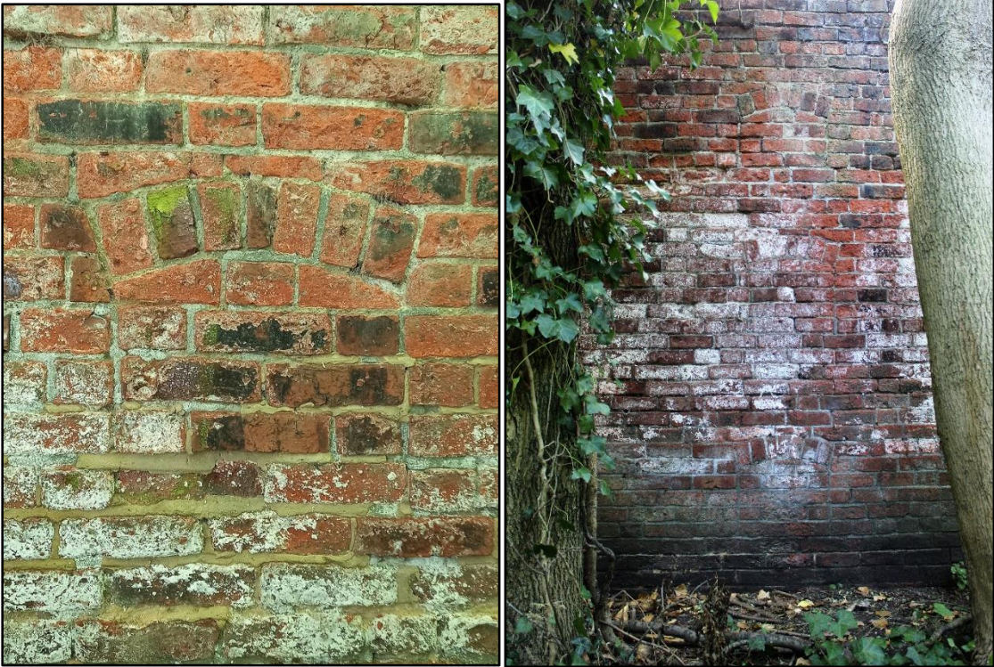
Fig 7 Blocked up flues in the north face of the Hot Wall. The image on the left shows an individual flue and the one on the right shows three flues, one above the other.
