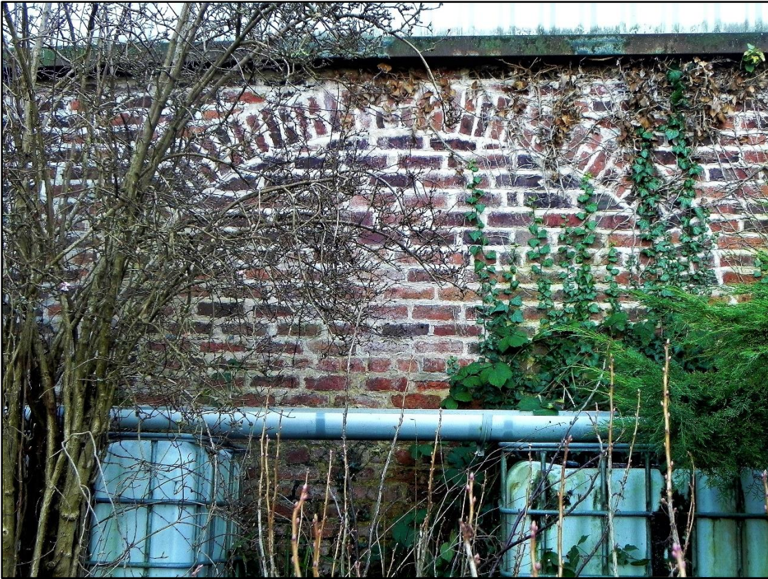
Fig 9 The blocked-up entrance in the south wall.
