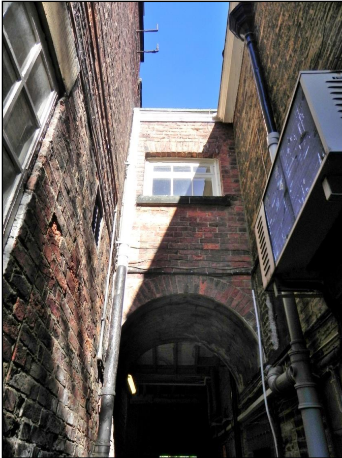
Fig 23 The brick bridge connecting the two structures.
